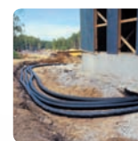
Flexibly and quickly through the brickwork to the main distribution point.
